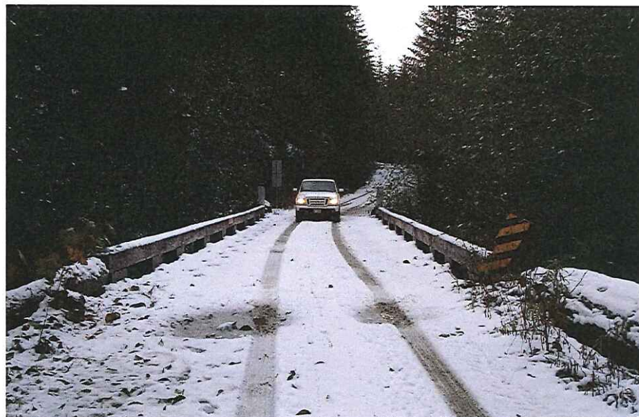
CK-2026 Approach Right Bank
