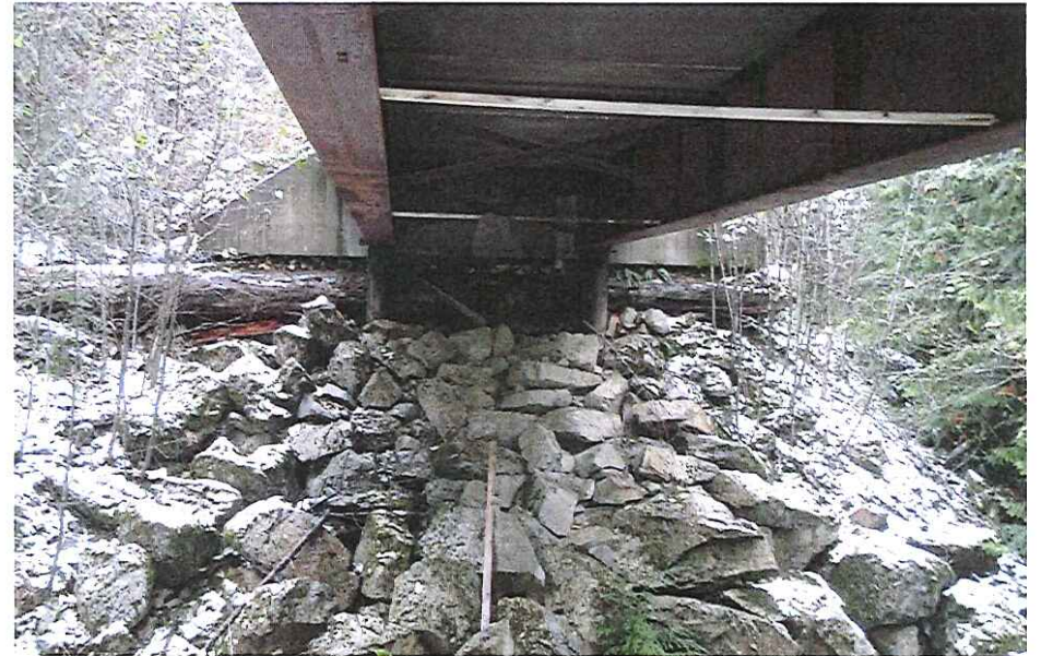
CK-2026 Abutment Left Bank
