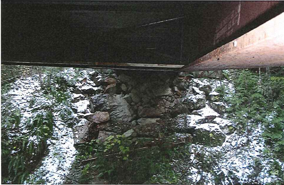
CK-2026 Abutment Right Bank
